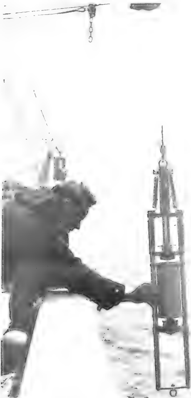
ABOARD THE ALBATROSS III --BIGELOW WATER SAMPLER READY TO BE LOWERED.
